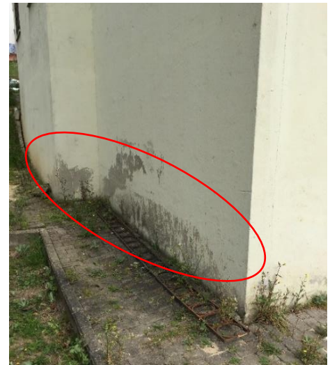
Fig.9 Type-1.1 efflorescence (northwest)
