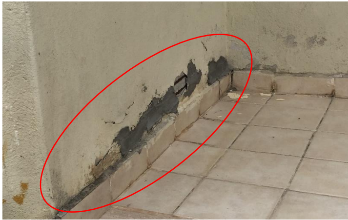
Fig. 34. Type-1.1 corrosion (northeast)
