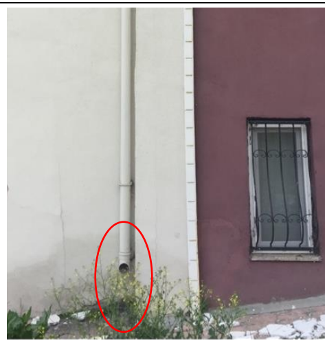
Fig.29. Type-2.1 rain downspout (northeast)
