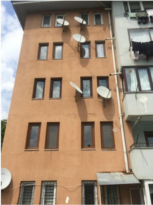
Fig. 22. Type-2.2 facade view (southeast)
