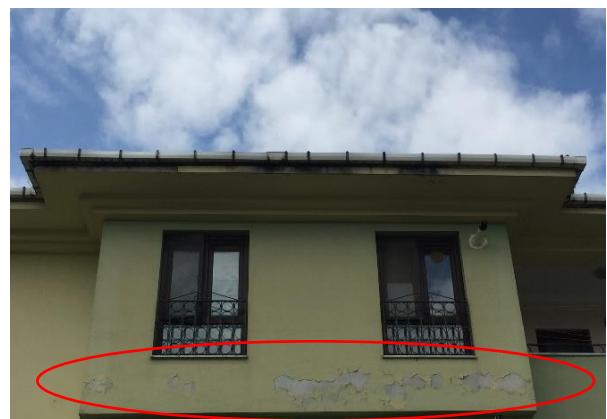
Fig. 15. Type-1.2 Paint damage (southwest)
