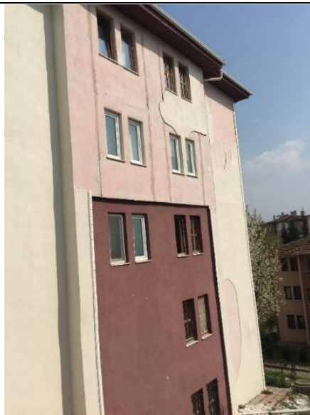
Fig.32. Type-2.1 Facade deterioration (southeast)
