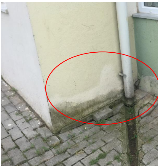
Fig.10 Type-1.2 Efflorescence (southeast)
