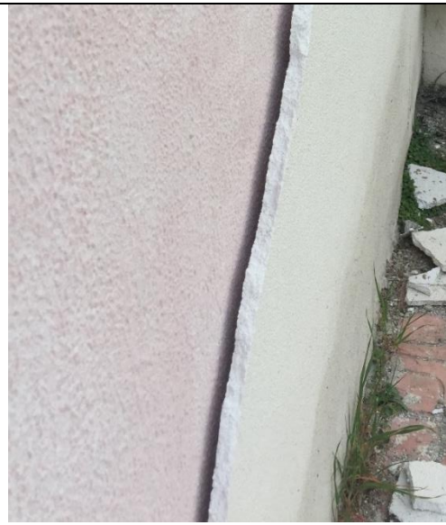
Fig 33. Type-2.1 Facade deterioration (southeast)
