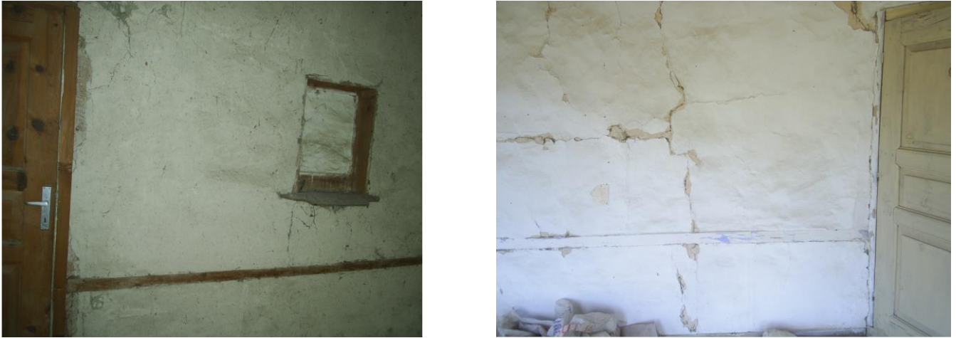
Figure 19. İbrahim Pilavcı House of wall views.
