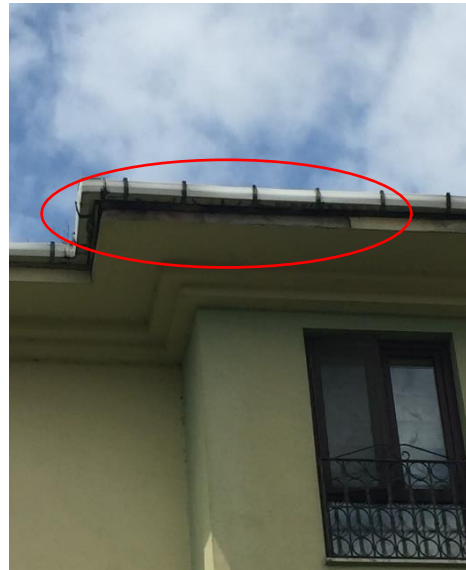
Fig. 17. Type-1.2 Corrosion on the roof (southwest)
