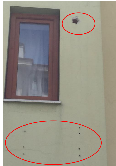
Fig.23.Type-1.2 anchor materials and drilled holes
