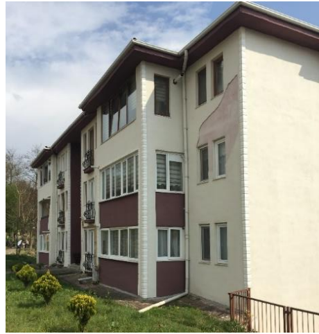
Fig. 31.. Type-2.1 facade deterioration
