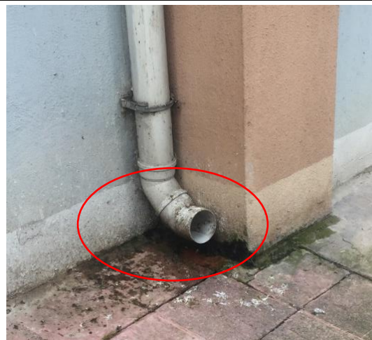
Fig. 27. Type-2.2 rain downpipe (northwest)
