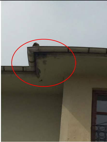
Fig. 16. Type 1.1 Corrosion on the roof (southwest)
