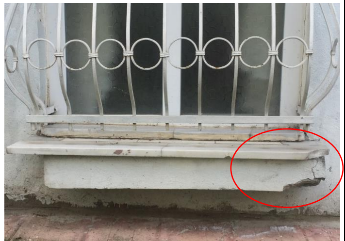
Fig. 19. Type-2.2 Wear in horizontal discharge (northeast)
