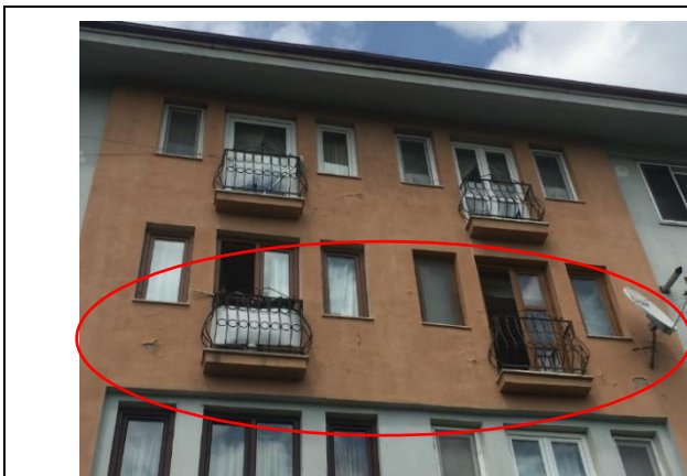
Fig.14 Type-2.2 Paint damage (southwest)
