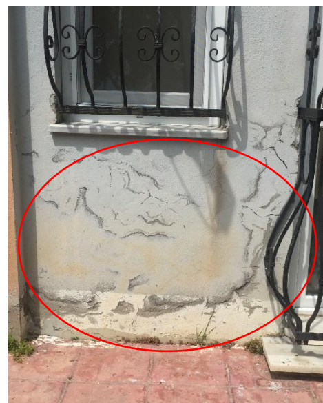
Fig.11 Type-2.3 efflorescence(northwest)
