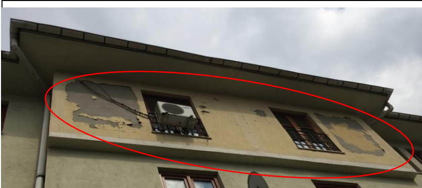
Fig. 12. Type-1.1 Paint damage (southwest)
