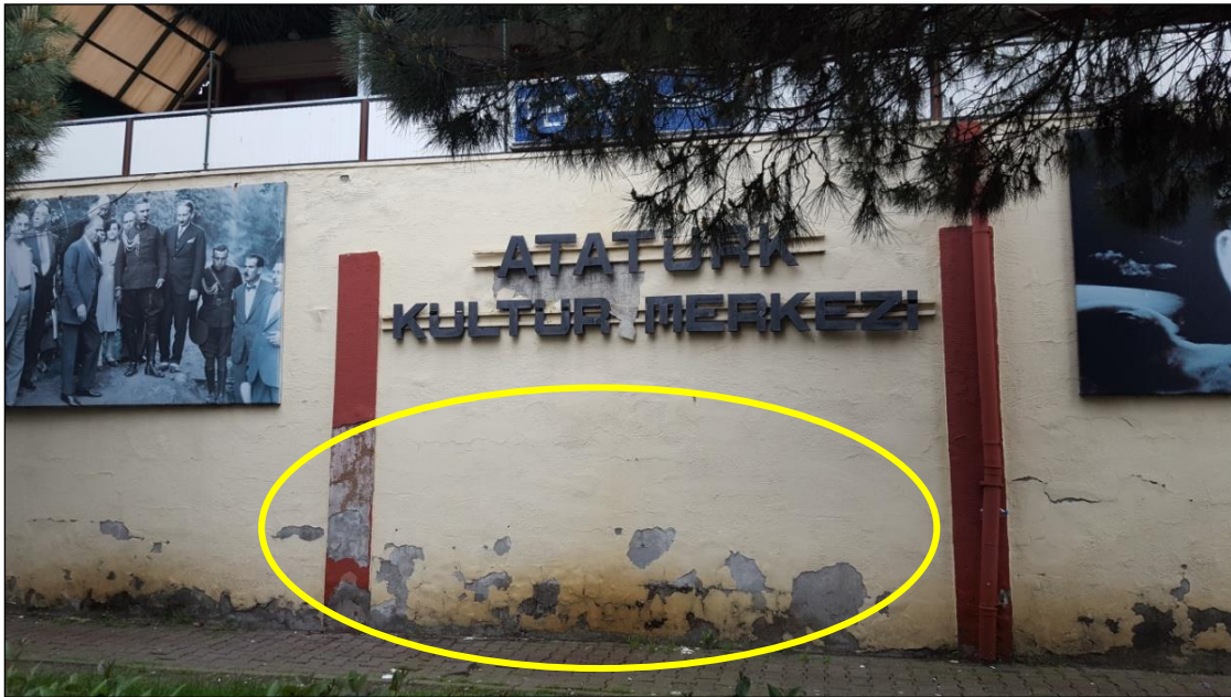
Photo 1. Damage to the facade exposed to water.
