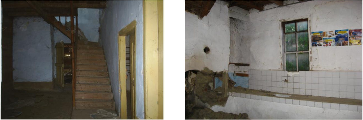
Figure 21. İbrahim Pilavcı House of stairs and ve kitchen views.
