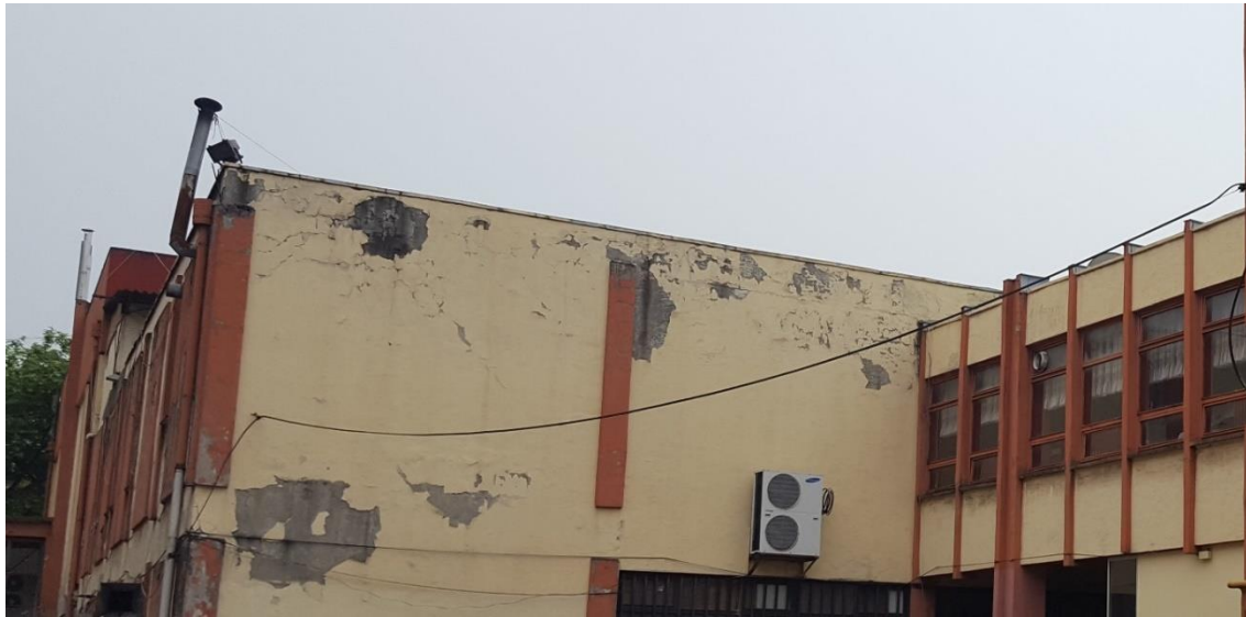
Photo 8. Damage to the facade exposed to rainwater
