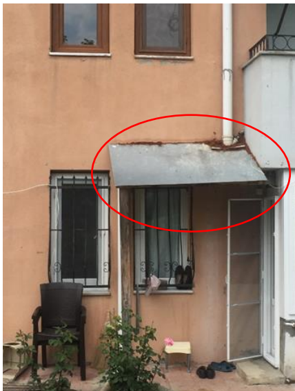
Fig.24. Type-2.2Eaves attached to the facade(southeast)
