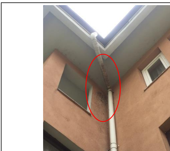
Fig.28.Type-2.2 Rain downpipe and bird droppings
