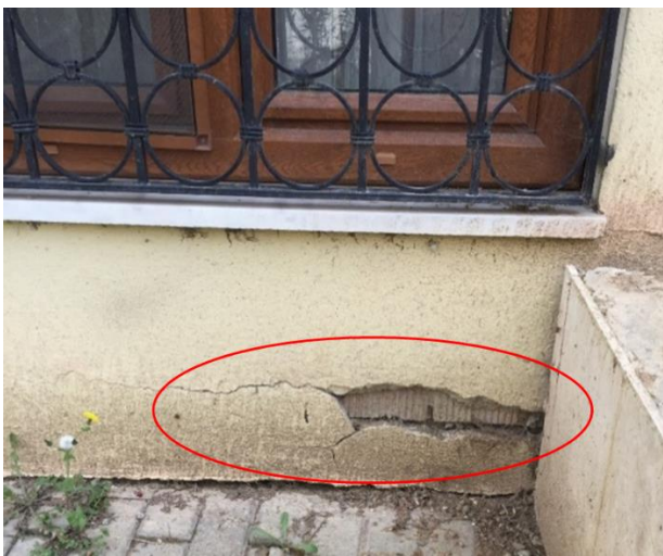
Fig. 18. Type-1.2 Wall surface corrosion (northeast)
