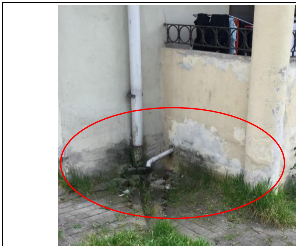
Fig. 26. Type-1.1 Rain downpipe (northeast)
