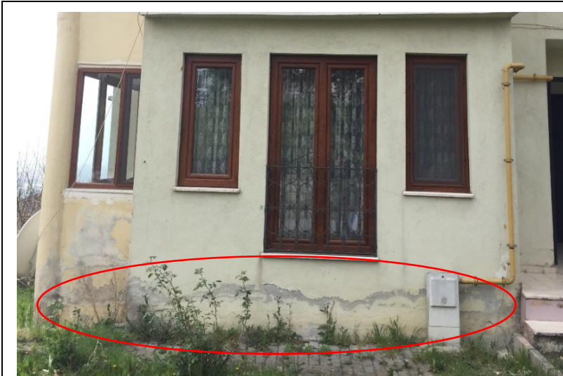
Fig.8 Type-1.1 efflorescence(northeast)
