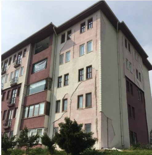
Fig. 30.. Type-2.1 facade deterioration
