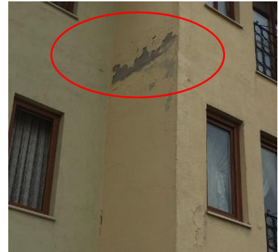
Fig.13. Type-1.1 Paint damage (northeast)
